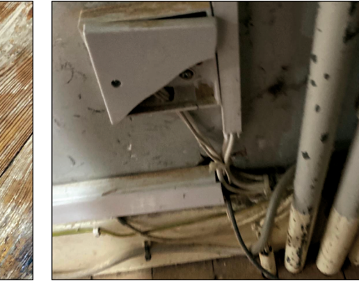
done in the Upper Hall, both on-stage and floorboards and dangerous electrical wiring
