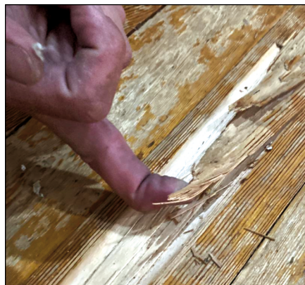
Examples of the work that needed to be done off-stage, included badly splintered floorboards.
